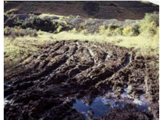
Driving in wet conditions quickly cuts up the track causing severe damage. Avoid driving in these conditions. Photo: Marcus Simons
